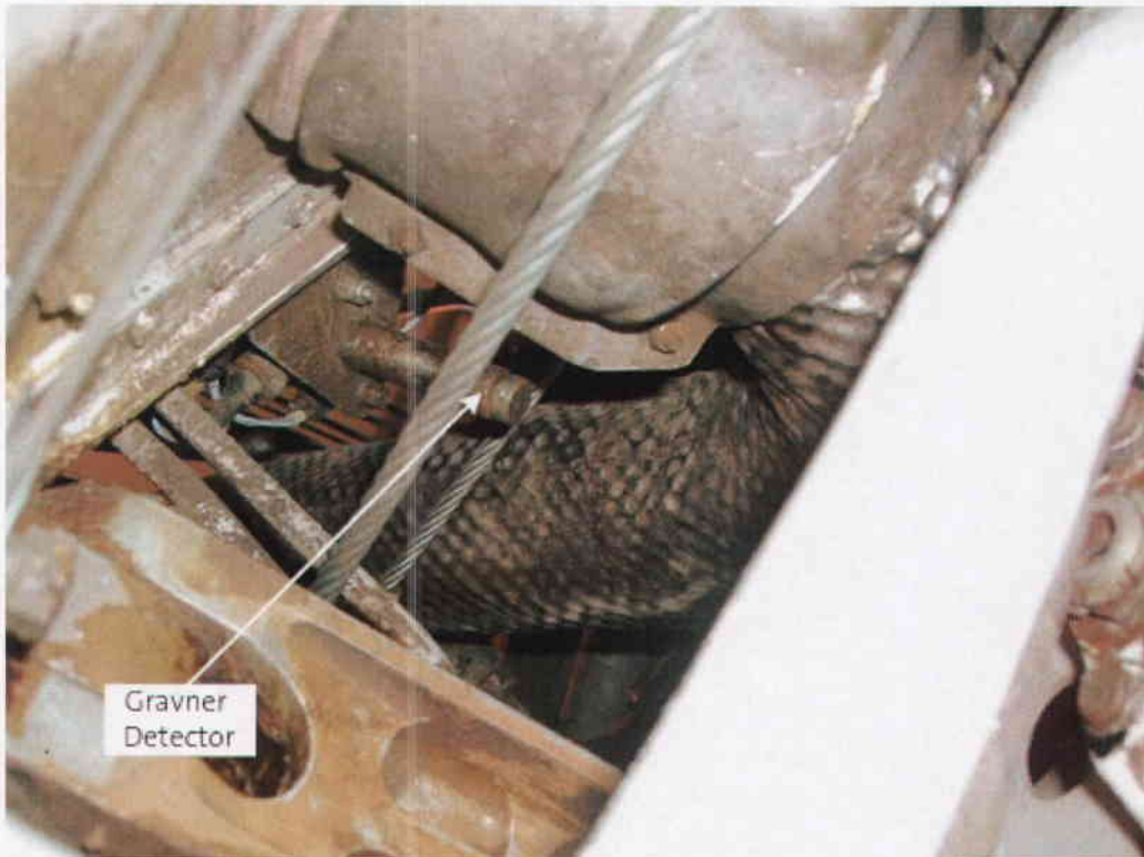
Figure 5 – Port Tank 7 Dry Bay (Bottom View)
